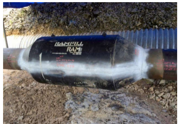
RAMFILL SLEEVE FULLY INSTALLED: WELDED, NDT INSPECTED & FILLED WITH RAM LIQUID EPOXY.
