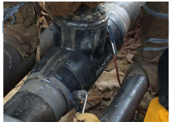
SLEEVE FITTED AND BEING WELDED
