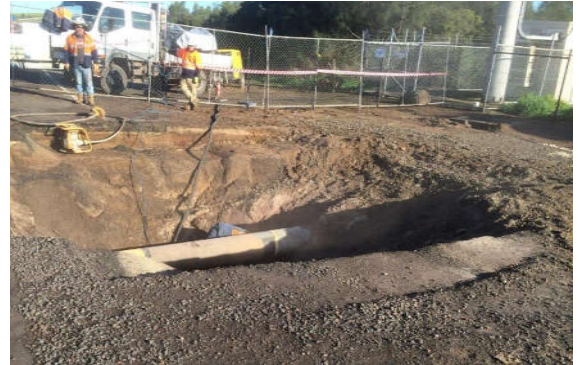
PIPELINE BEING GRIT BLASTED
