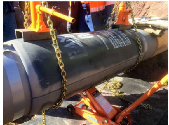
SLEEVE FIT-UP PRIOR TO WELDING
