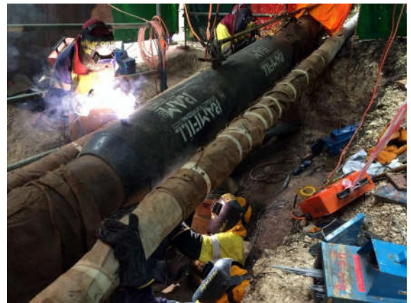
CLOCK SPRING WAS APPLIED, AT THE TIME, AS AN EMERGENCY REPAIR.
