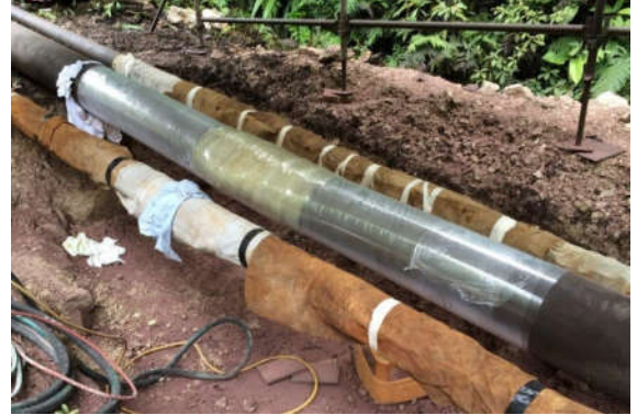
CLOCK SPRING WAS APPLIED, AT THE TIME, AS AN EMERGENCY REPAIR.
